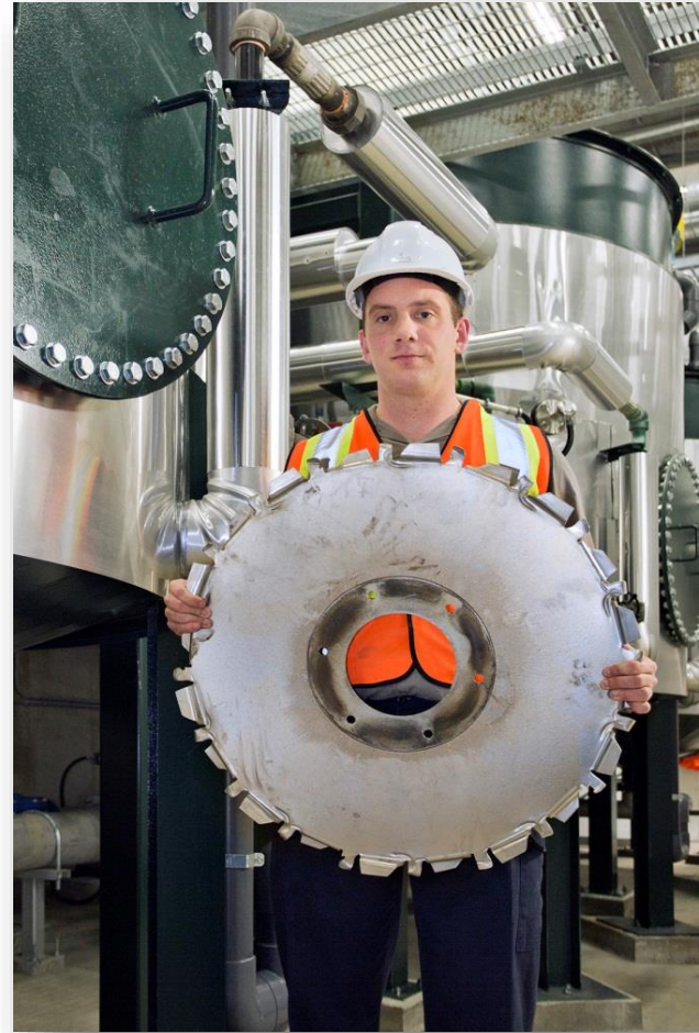
Process reactor & high speed shearing blade
